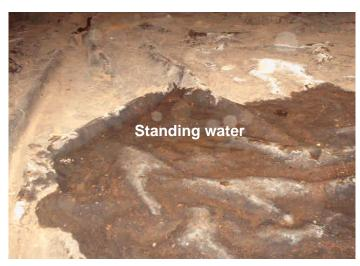
2.13 - There is evidence that moisture is migrating through the walls of the foundation. The moisture is intruding through gaps in the seam between the foundation wall and the footing. This is not unusual. We recommend sealing the gaps with an appropriate caulk or grout to help prevent further moisture intrusion.
